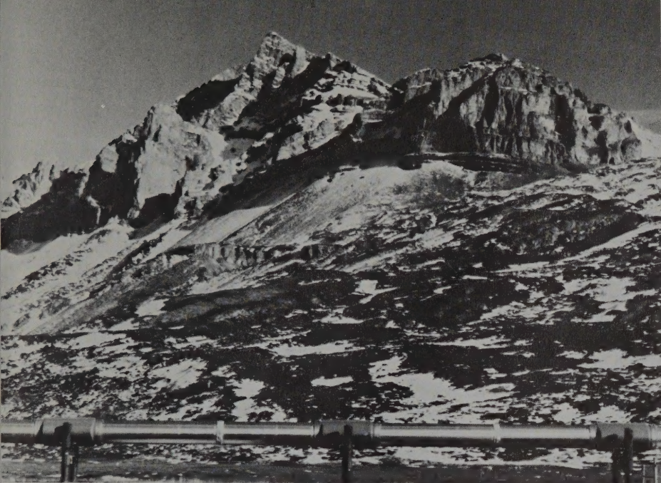
The 48-inch, insulated pipeline traverses rugged country to bring oil from the arctic.
